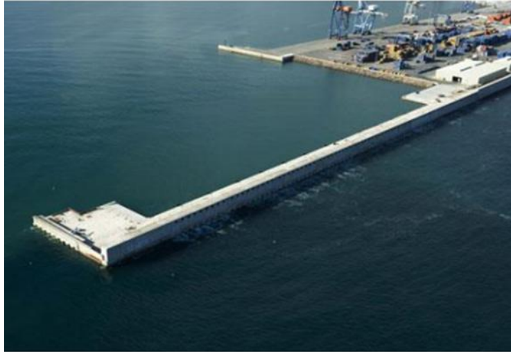
Fig 2.4: Vertical breakwaters
