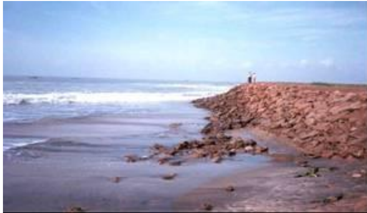
Photo 5.4 Single Layer Armour Revetment
