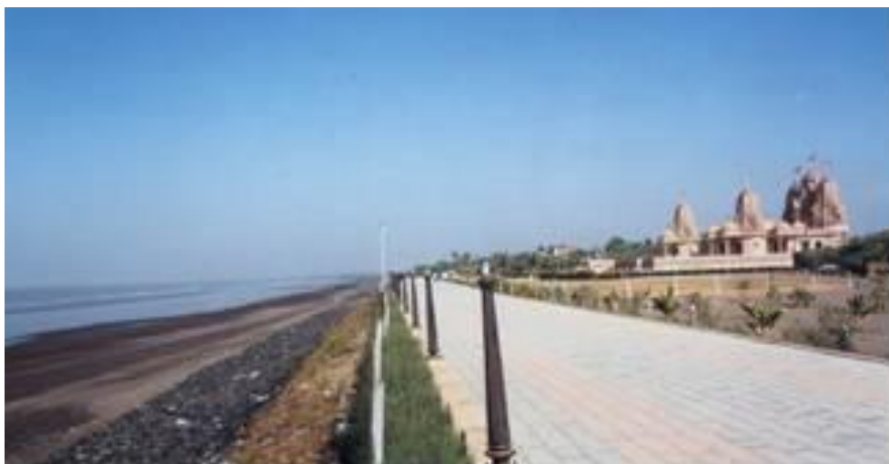
Photo 5.6 Well Maintained Seawall
